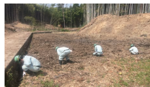
Original design (full improvement) Design change (halved the scope of improvement to secure groundwater permeability) Gaps are left in the improve part An example of water scorpion ( Nepa hoffmanni ) conservation
