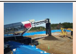
Interim storage facilities, soil storage facilities
