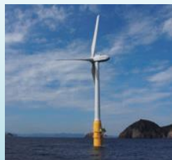
Offshore wind power generation facility (from Annual Report on the Environment 2016)
