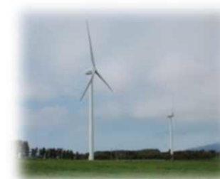
Wind power generation (from MOEJ website)
