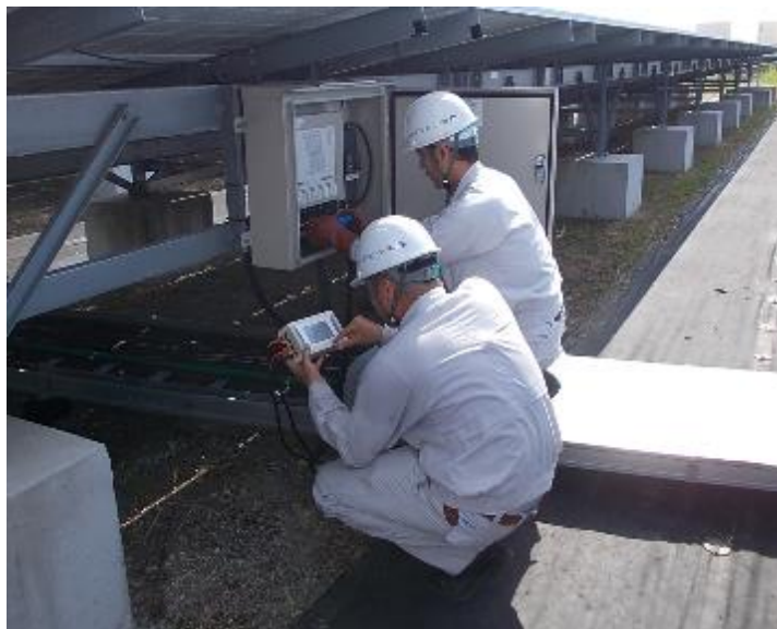
Reference picture taken during I-V inspection (example of on-site inspection)
