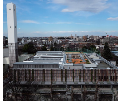
Waste treatment facilities as local energy centers and emergency centers
