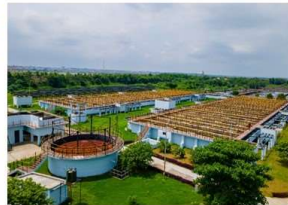
Rajapur , Prayagraj 90 MLD NJK (STP)
