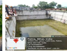
Maner, Patna 6.5MLD NJK (STP)
