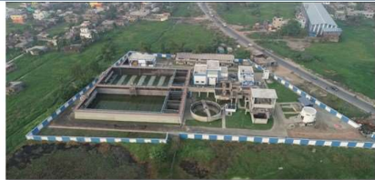
Barrackpore 24 MLD NJK (STP)
