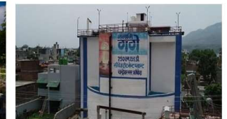
Chorpani 7.5 MLD NJK (STP)
