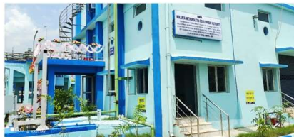
Budge Budge 9.3 MLD NJK (STP)
