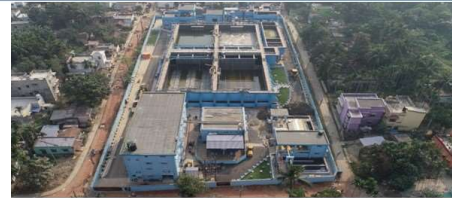
Halishahar 16 MLD NJK (STP)
