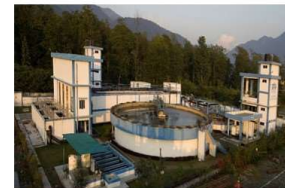
Chorpani, Muni Ki Reti 5 MLD NJK (STP)
