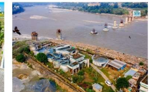
Srinagar 3.5 MLD NJK (STP)
