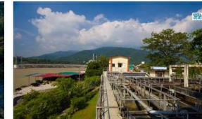
Rishikesh (Swargashram) 3 MLD NJK (STP)
