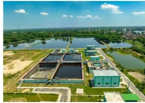
Masani, Mathura 30 MLD NJK (STP)
