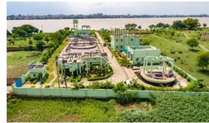
Ramnagar , Varanasi 10 MLD NJK (STP)
