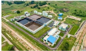
Ramanna , Varanasi 50 MLD NJK (STP)
