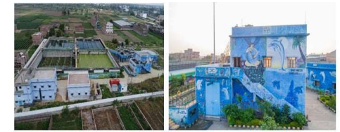
Karmalichak, Patna 37MLD NJK (STP)
