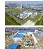
Example of PFI (Resource Recovering Project (Power generation and carbonized fuel production) in Toyohashi City)
