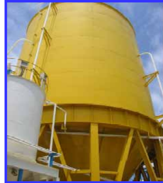
Anaerobic digester
