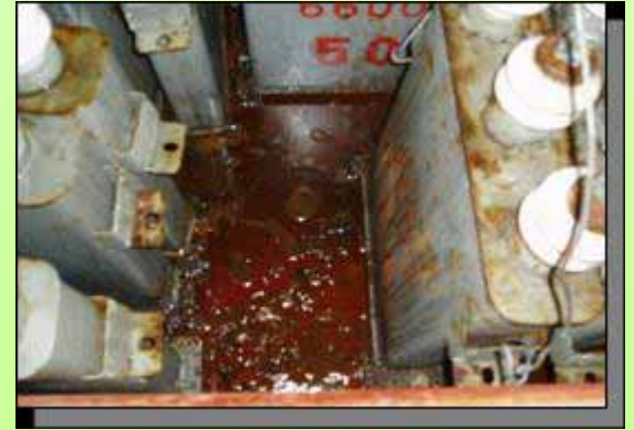
[Improper storage of PCB waste]
