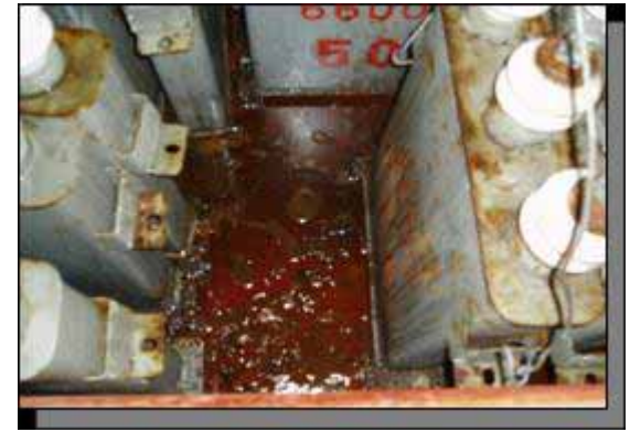
[Improper storage of PCB waste]
