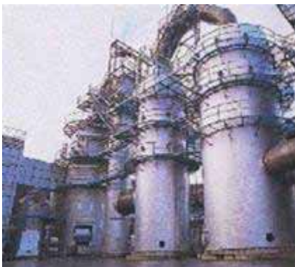
Plant for recovery of rare metals
