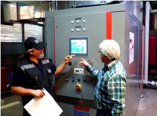
CHP plant in Chilean hospital; Credits: GIZ
