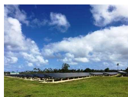
Photovoltaic panel introduced by Grant aid (Tonga)
