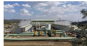
Geothermal Power Plant introduced by ODA Loan (Olkaria · Kenya)
