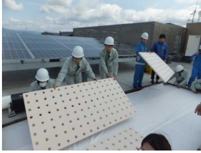
Working on the rooftop
