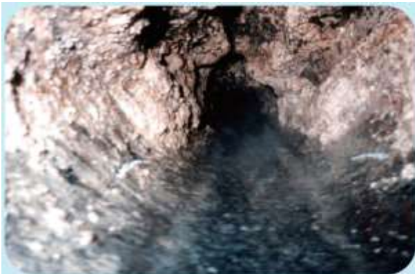
Sewer pipe is clogged up with oil
