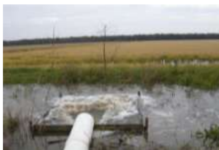
Pic9. Silt basin and screen.
