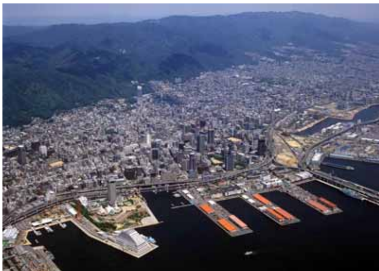
Picture: A cross shot of the Rokko Mountain Range and the urban district at the bottom of the mountains (Source: Brochure by Rokko Sabo Works Office, Ministry of Land, Infrastructure and Transport, “Rokko Mountain Range Green Belt Development Project”)
