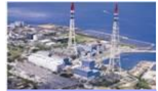
Makiminato Thermal Power Station
