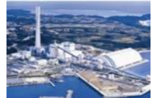
Kin Thermal Power Station
