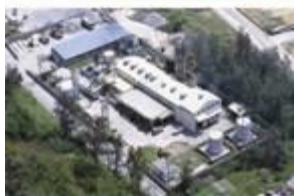
Tokashiki Power Station
