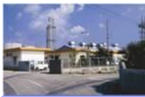
Kitadaito Power Station
