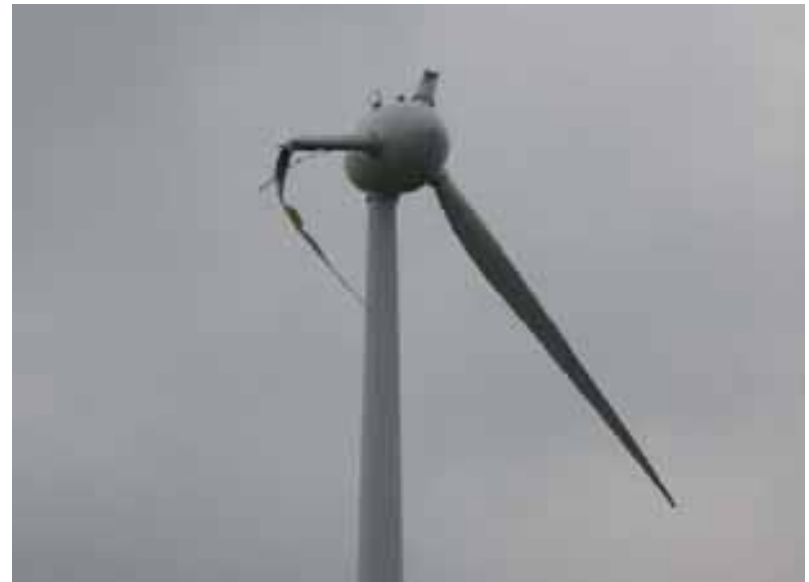
Yonaguni No.1 (Damaged in Typhoon No. 15 in 2007)
