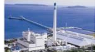
Gushikawa Thermal Power Station
