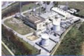
Kumejima Power Station
