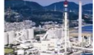
Ishikawa Thermal Power Station
