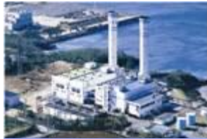
Miyako No.2 Power Station
