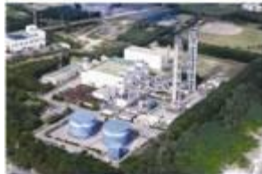
Ishigaki No. 2 Power Station
