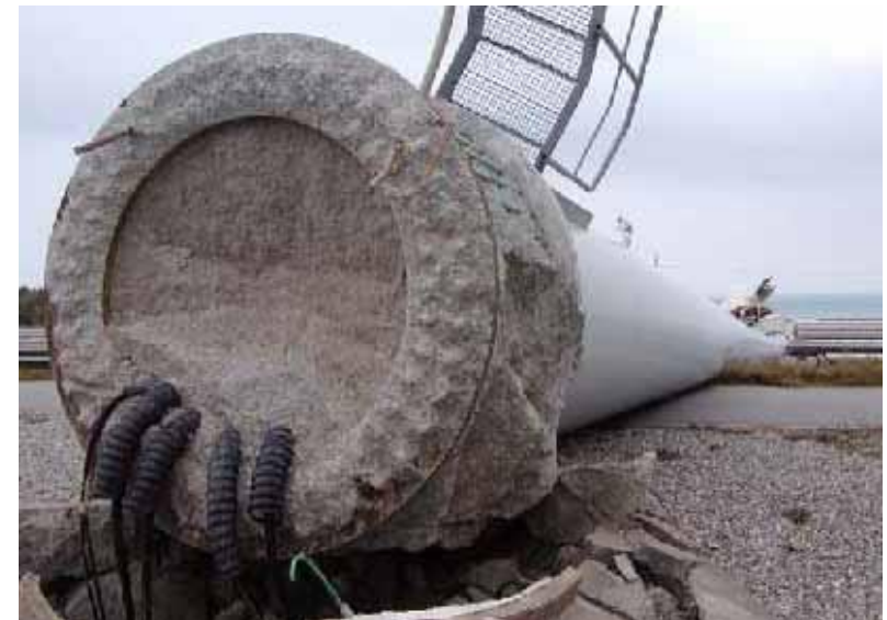
Miyakojima Nanamata No.1 (Damaged in Typhoon No. 14 in 2003)
