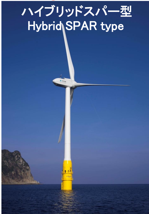
環境省浮体式洋上風力発電実証事業 Ministry of the Environment / Floating Offshore Wind Turbine Demonstration Project Small- scale Test Plant
