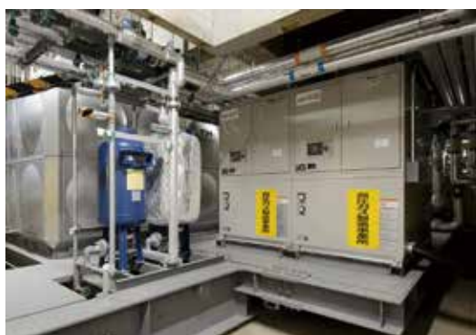
Heat recovery type heat pump
