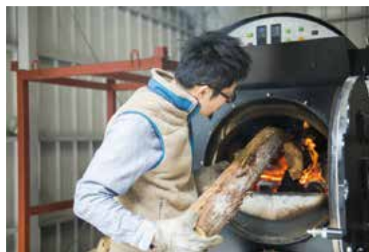
Wood-fired boiler for hot spring facilities
