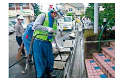
Removing sludge in street gutters (photo: Fukushima City)
