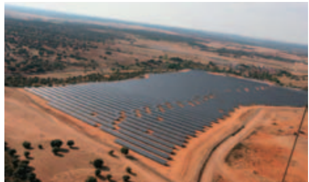
Planta Solar de Salamanca, a large scale PV power generation facilities in Salamanca, Spain (facility area: approximately 360,000m 2 ) (Photo: courtesy of KYOCERA Corporation)
