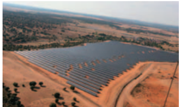
Planta Solar de Salamanca, a large scale PV power generation facilities in Salamanca, Spain (facility area: approximately 360,000m 2 ) (Photo: courtesy of KYOCERA Corporation)
