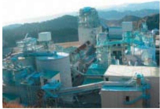
A picture of an eco-cement plant Source: the homepage of the Tokyo Tama Extended-area Resource Cycle Cooperative
