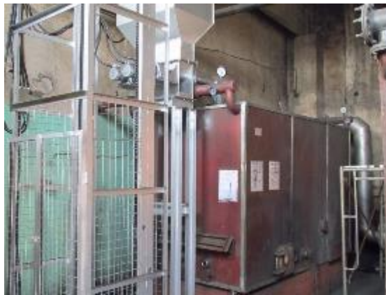
Coal supply system
