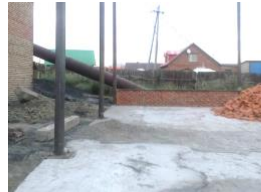
Construction of floor
