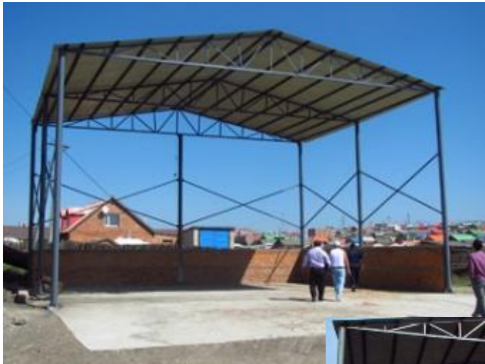
Complete view of coal storage site
