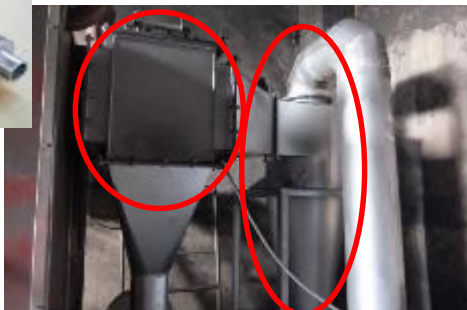
Air heater, left, and cyclone, right
