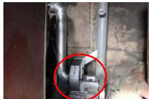
Induced draft fan
