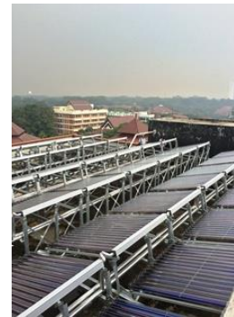
Installed heat collector
