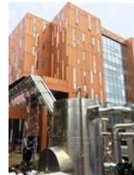
Schoolhouse with equipment installed
