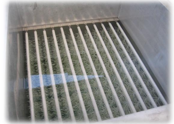
Swim bed installed inside a tank
