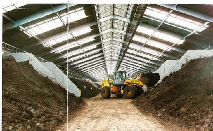
Figure E.1 Fermentation building
