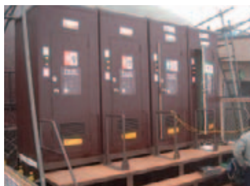
[Waste water treatment in mountainous areas] Source : Ministry of the Environment
