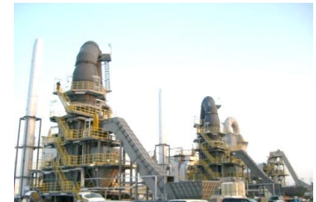
Temporary incinerator in Souma city, Fukushima (2013.1.16)
