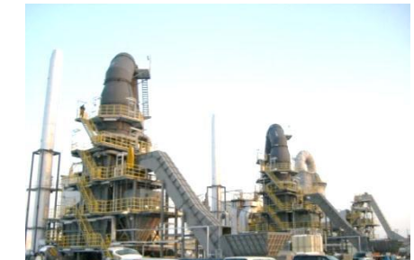
Temporary incinerator in Souma city, Fukushima (2013.1.16)
