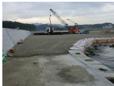
Shizugawa fishing port south-side breakwater restoration work
