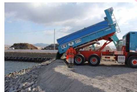
Ishinomaki Port embankment project (Landfill started on Feb.20, 2013)
