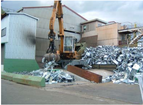
Collecting the Scraps by Excavator (Source: Consultant Document)
