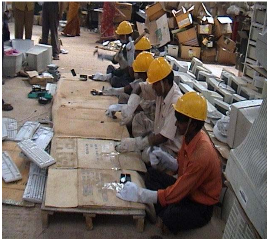
Controlled Dismantling Activity
