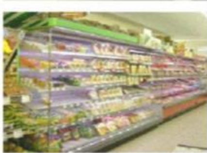
Refrigerated display cabinets connected with centralised cooling station
