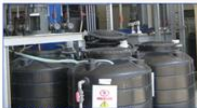
Waste Water Treatment Plant
