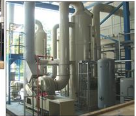
Counter-Flow Wet Scrubber System
