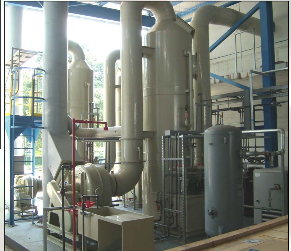
•Counter-Flow Wet Scrubber System
