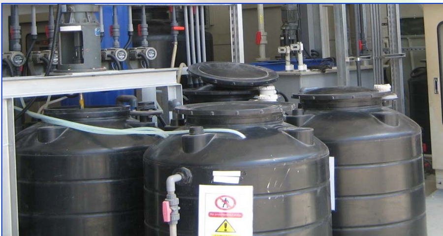
•Waste Water Treatment Plant
