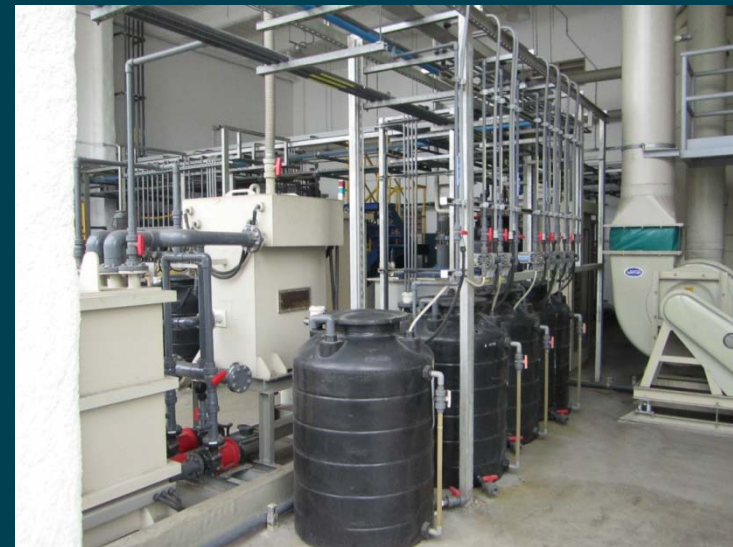
Waste liquid treatment facility
