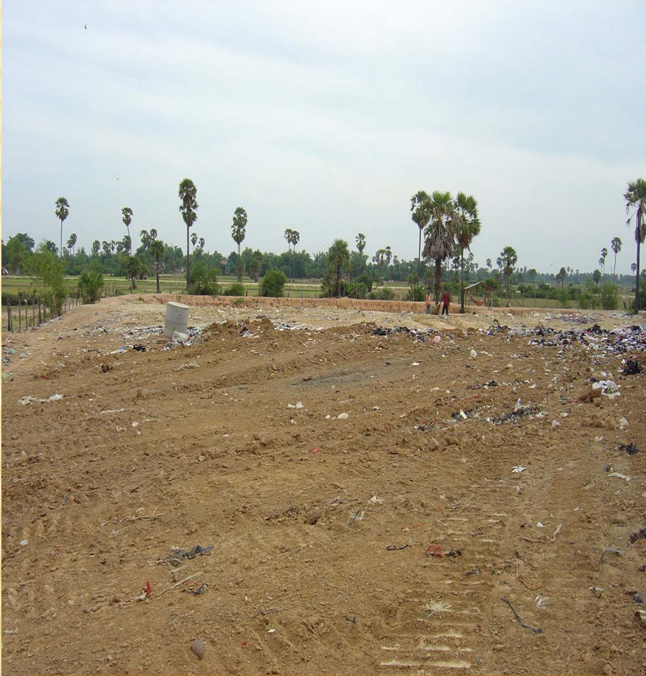
Landfill closed and soil covered
