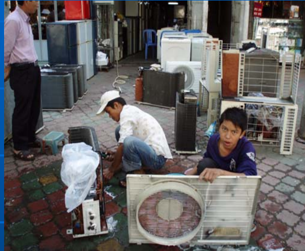
Pic. 22: Impractical repairing of air-con by local fixers, Kandal Province
