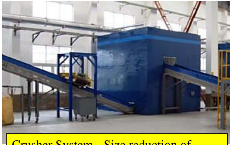
Crusher System - Size reduction of materials, Magnetic separation
