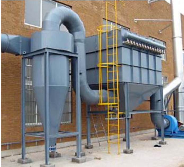
Dust collection system
