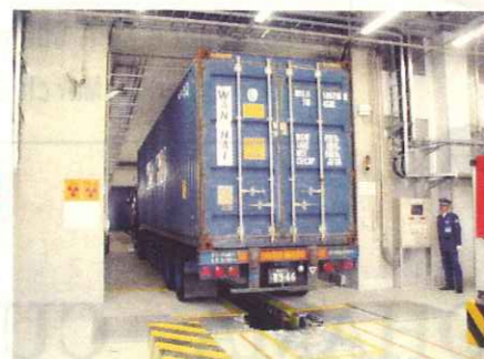
④ After the container is carried to the center of the X-ray machine, the shield door is closed and irradiation of X-ray is starts.
