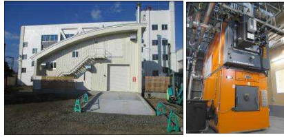
Wood biomass boiler in the Town Center
