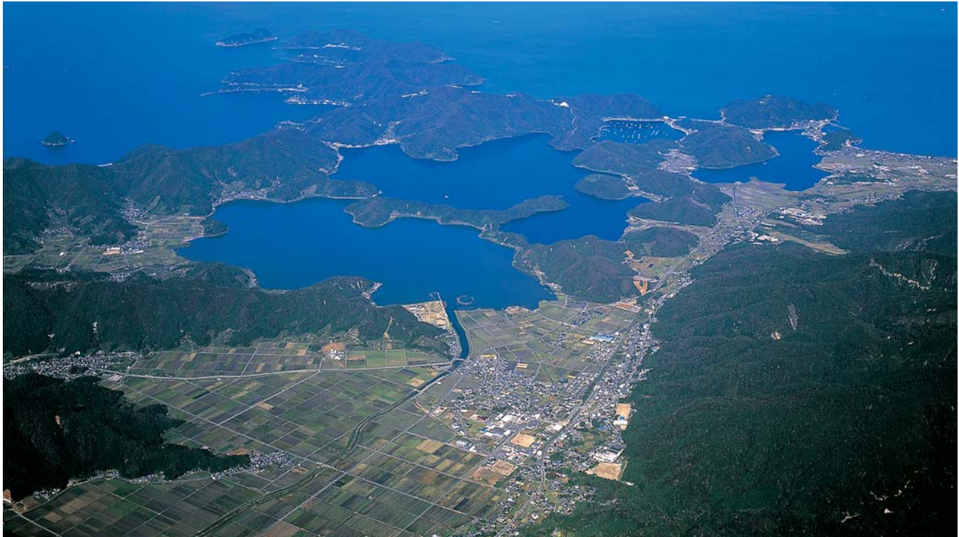
Aerial view of Mikata-goko from the south
