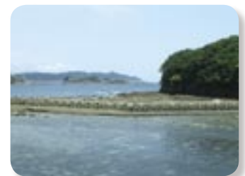
An existing breakwater levee
