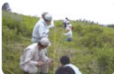
Protected vegetation zone and fence installation
