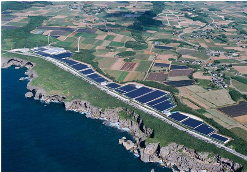
Mega Solar Site at Fukuzato, Miyakojima
