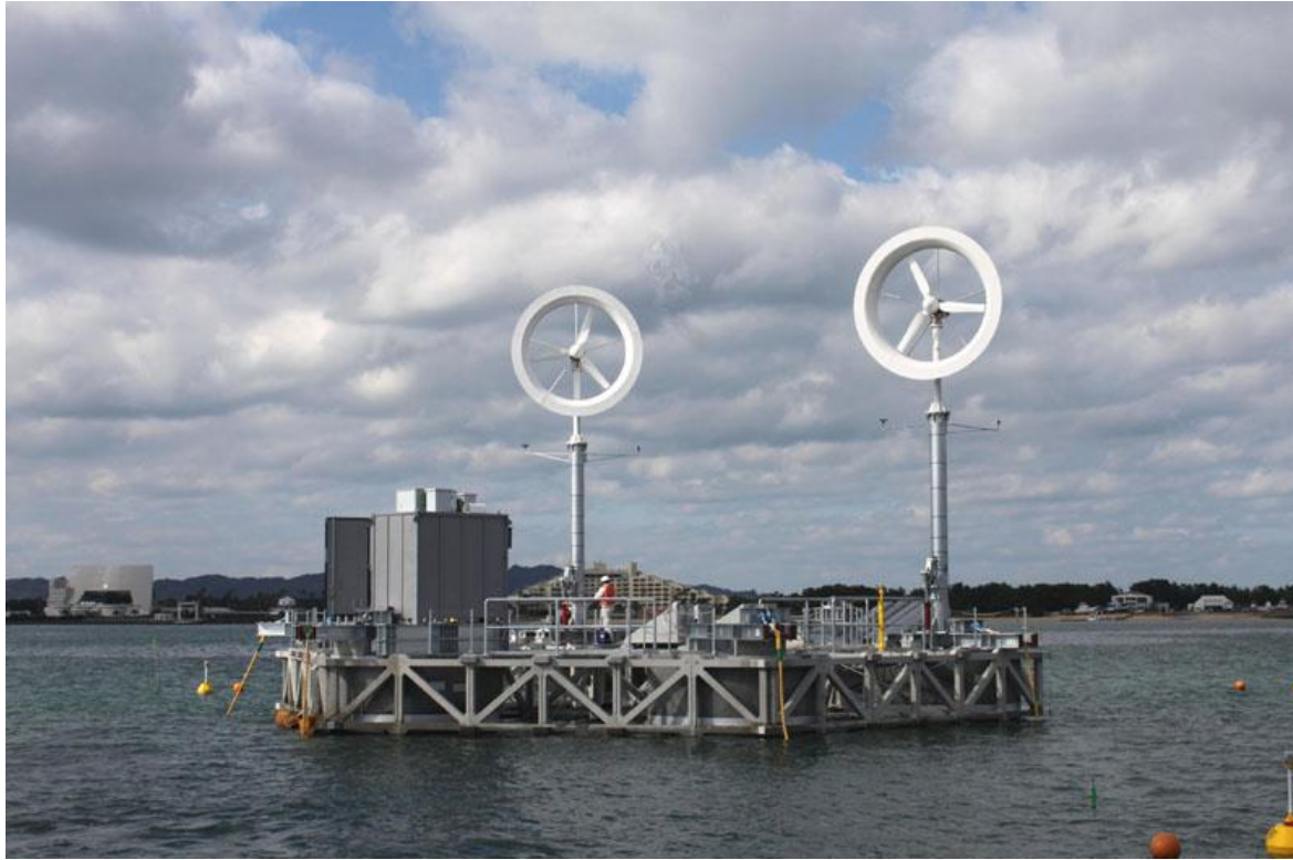
Wind turbines with wind diffusers on a float in Hakata bay, Fukuoka, Japan
