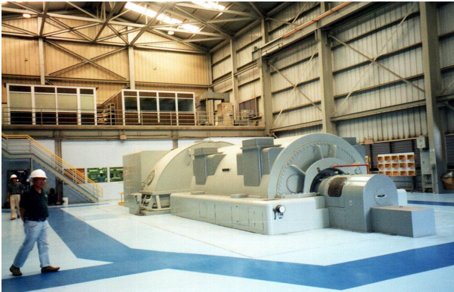
Power Generation by Waste Heat (Covanta, Honolulu)
