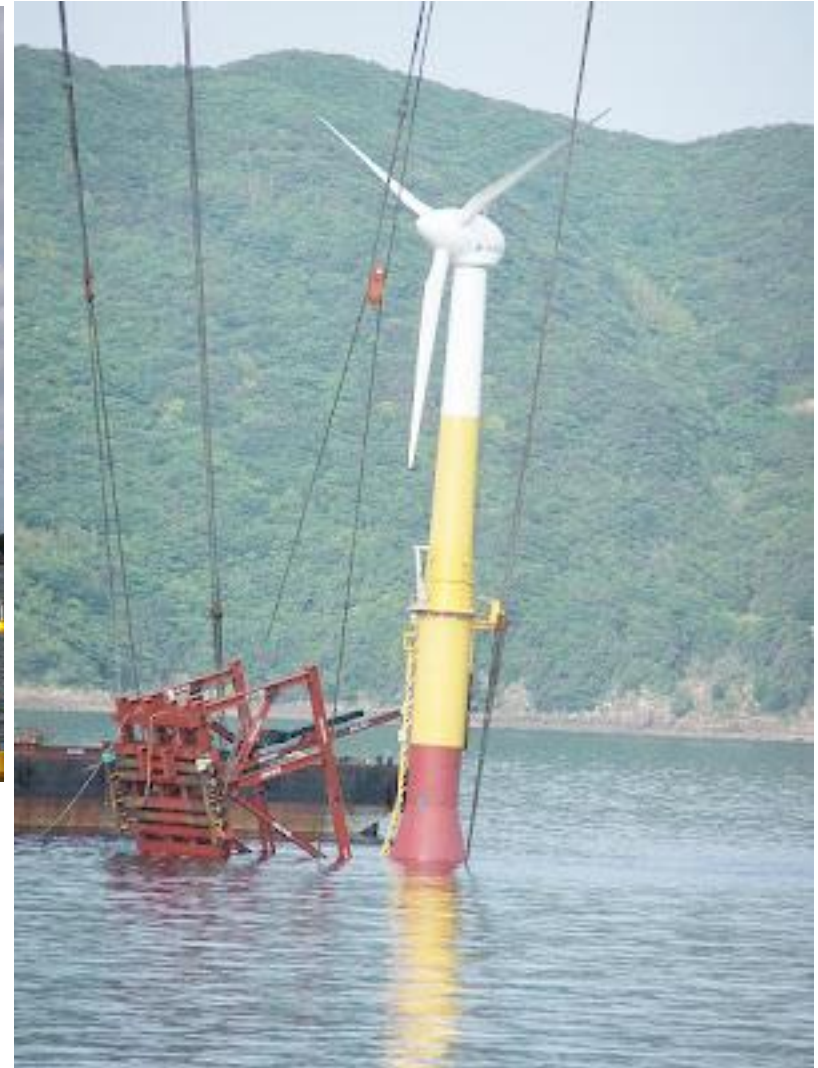
Test of a Self-float type wind turbine, Goto-City, Japan
