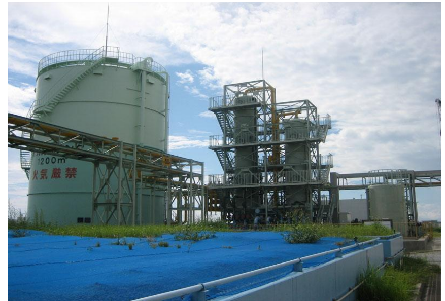
Power Generation by Bio Methane (Naha, Okinawa)
