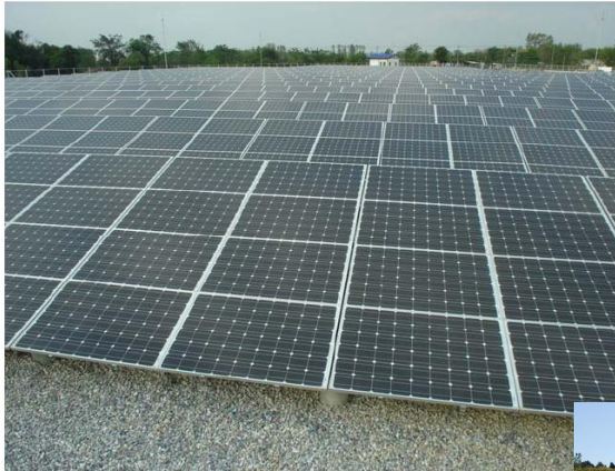
Solar PV Farm 35 MW
