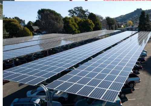
Solar PV Rooftop 50 MW
