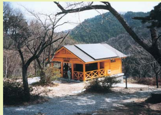
Refurbished restrooms (Chazonobara, Daisen-Oki National Park, Tottori)
