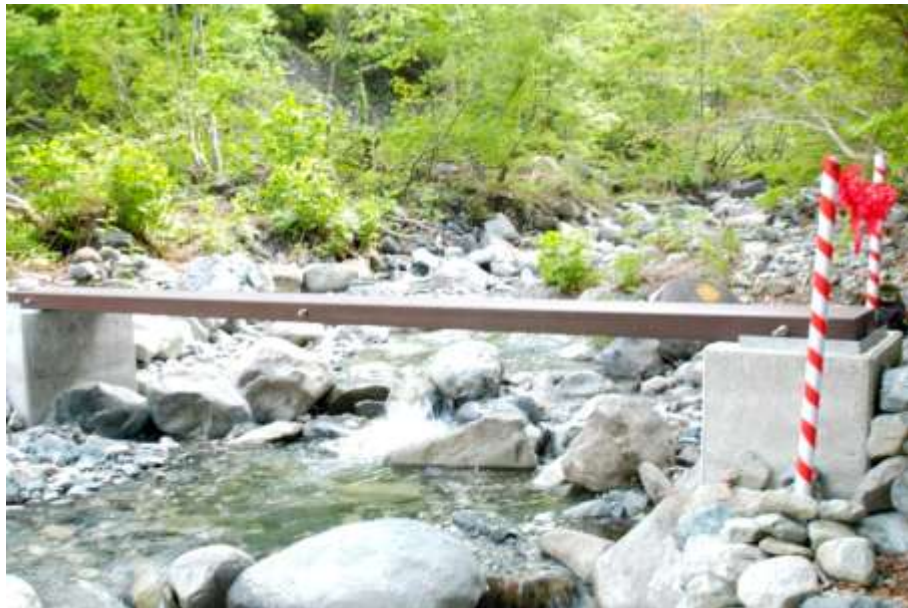
A Removable Bridge at Ichinokurawasa
