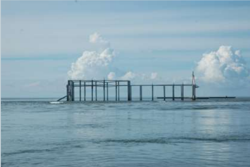
Evidences of land subsidence around Singkil after Nias earthquake in March 2005.
