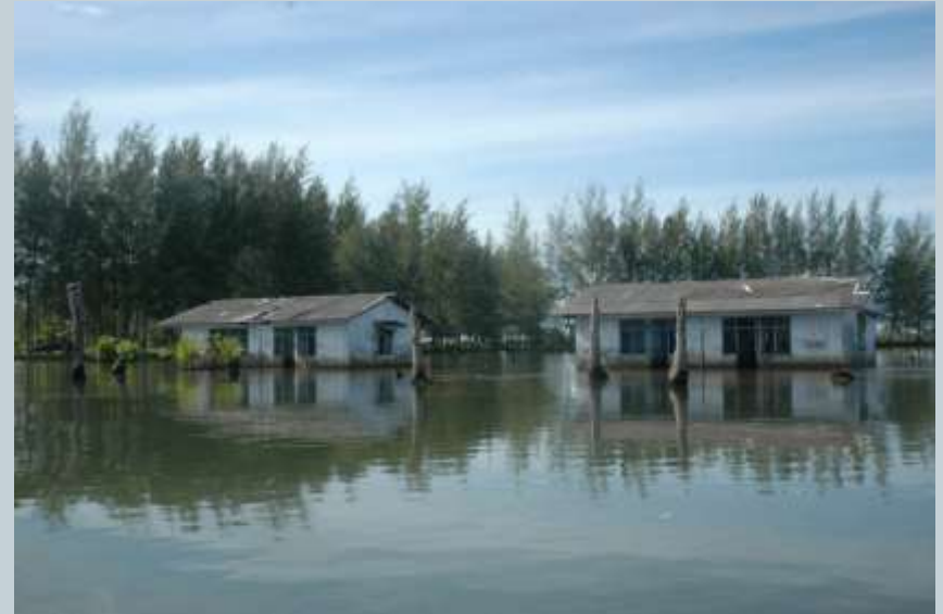
Evidences of land subsidence around Singkil after Nias earthquake in March 2005.
