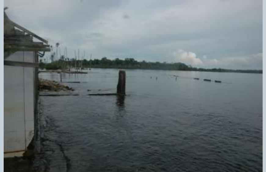
Coastal erosion at Haloban Island of Banyak Islands
