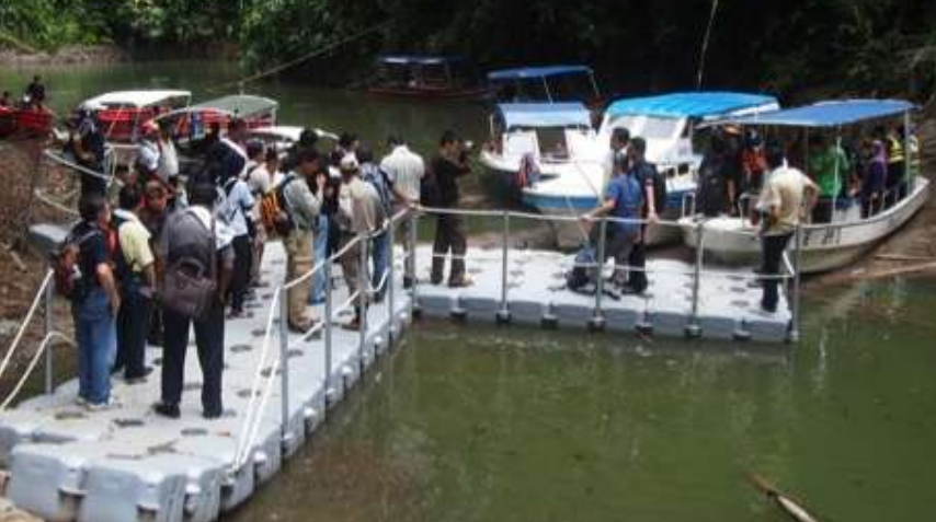
New pontoon jetties provided at Royal Belum State Park, Malaysia to boost visitation
