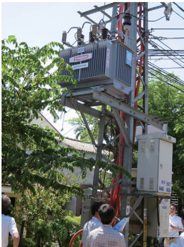
Amorphous Transformer Installed in Ben Tre Province
