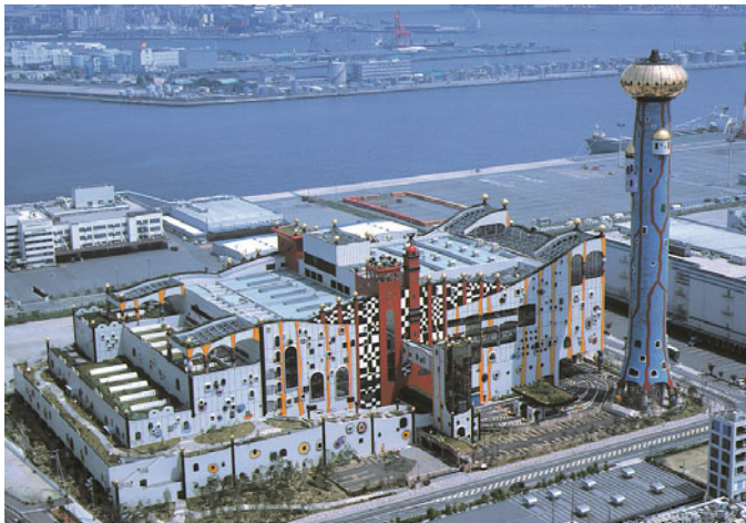
Osaka City Maishima WtE Plant constructed by our corporation
